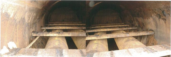
The scale is loose and no pitting is evident beneath. The horizontal supports appear to be securely attached to the heater shell and have no distortion.
