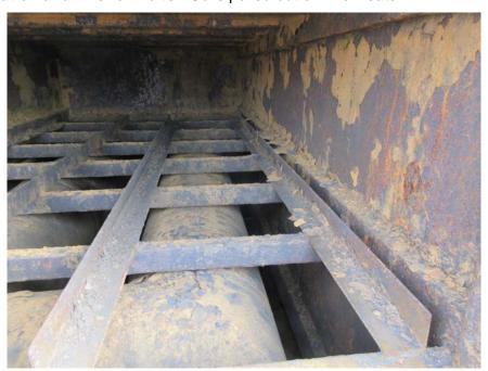
Condition of Steel Supports, Saddles and Bolting: (2) vertical plates have heavy surface corrosion and peeling.
