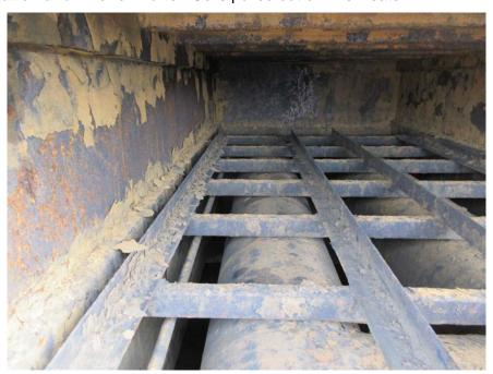
Condition of Paint and/or Insulation: Front plate has minor chipping with surface corrosion.
