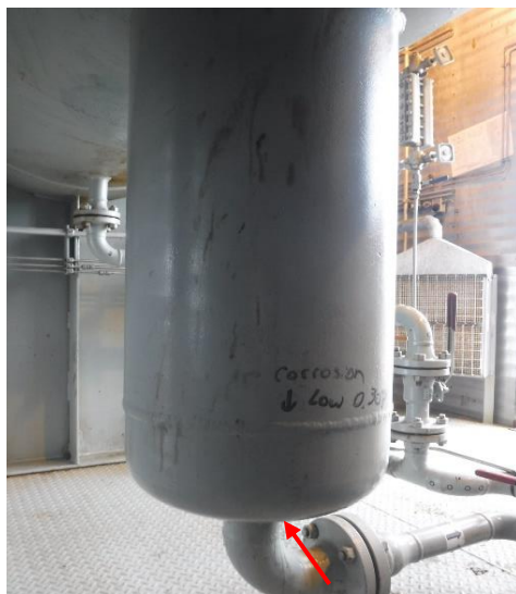
CORROSION ON EAST SIDE BOOT HEAD.
