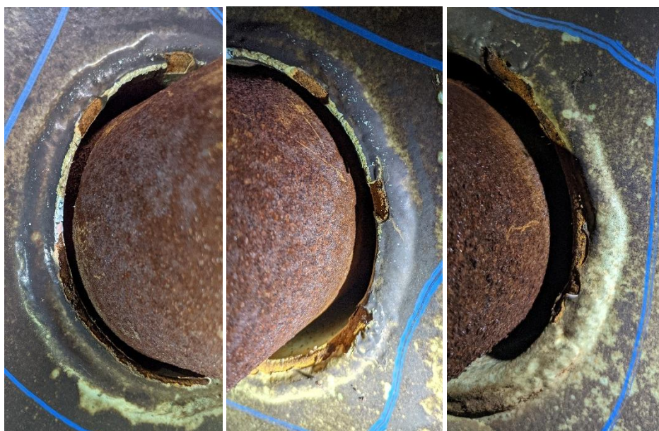
Figures 11 to 13 – Coating Holidays on the Level Column Nozzle
