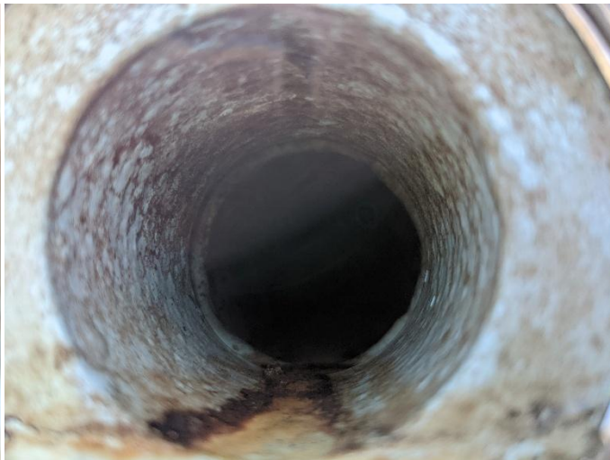
Figures 4 and 5 – 1.5" Nozzle Overviews from the Vessel Exterior Note: Left photo is of the left nozzle, right photo is of the right nozzle
