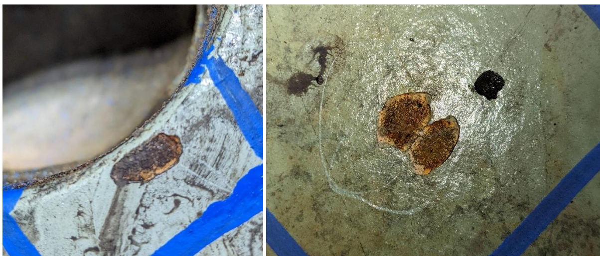
Figures 9 and 10 – Coating Holidays on the Bottom Shell, Near Drain Nozzle
