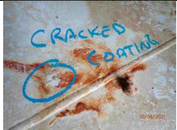
RARE-ST82253-AST-PrePurchase-Int-Overview1c-Coating Crack Closeup-10-06-2021.JPG
