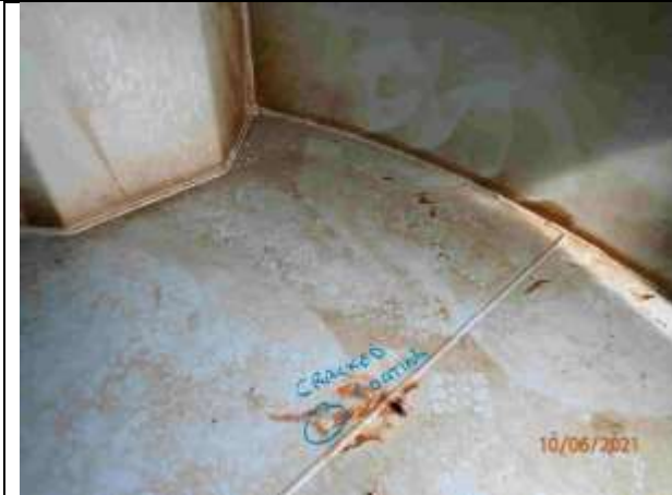
RARE-ST82253-AST-PrePurchase-Int-Overview1a-Coating Crack Overview-10-06-2021.JPG
