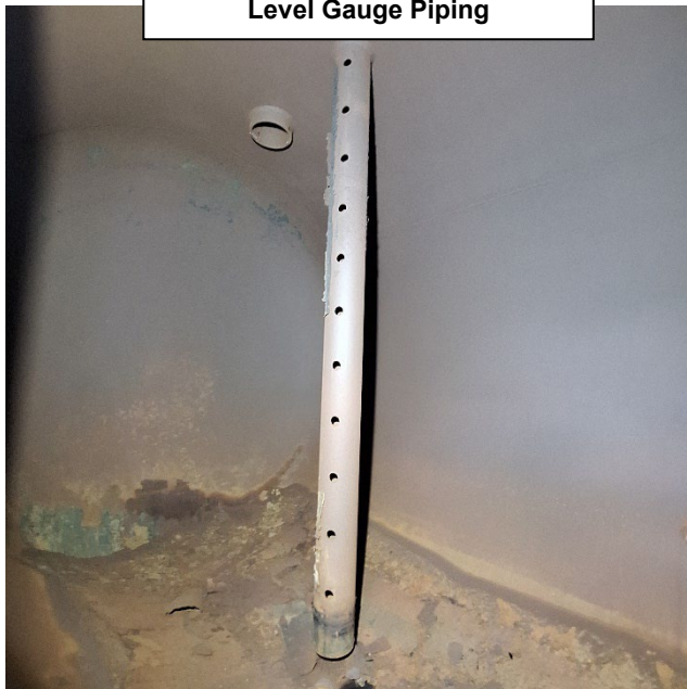
Level Gauge Piping
