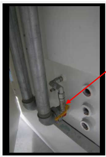
Figure 23 - A -Draining fluid details - Container installation
