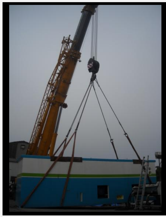
Figure 14 - Reinforced concrete hoisting example with crane
