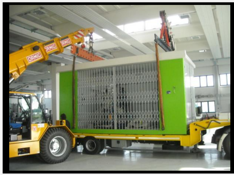
Figure 16 - Container hoisting and moving during delivery operation
