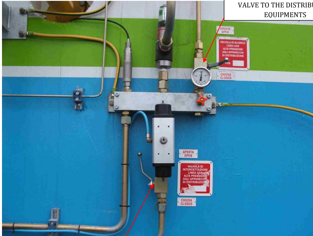
Figure 7 - B - Interception and unloading manual valves
