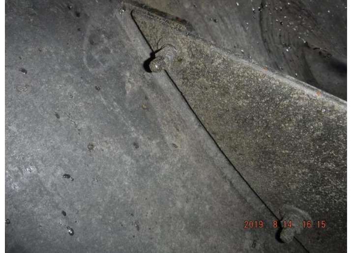
Typical Weir Bolting
