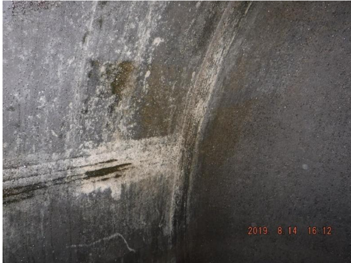
Rear Head to Shell T-Joint
