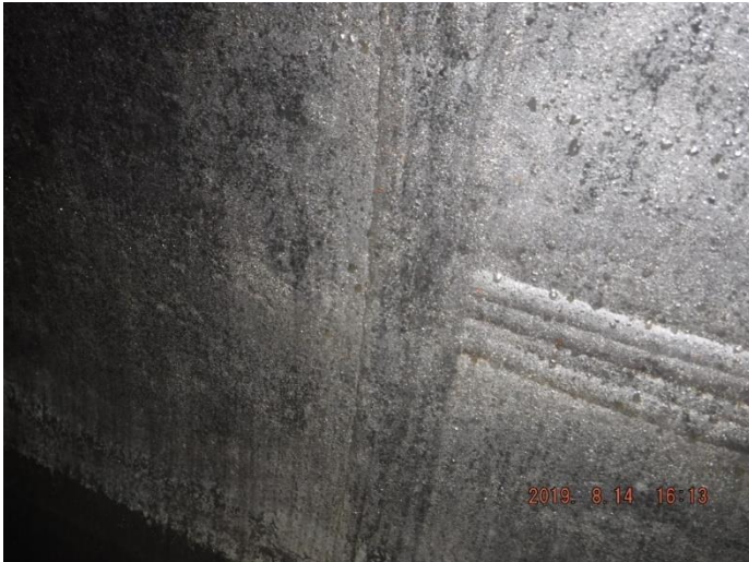
Typical Shell T Joint
