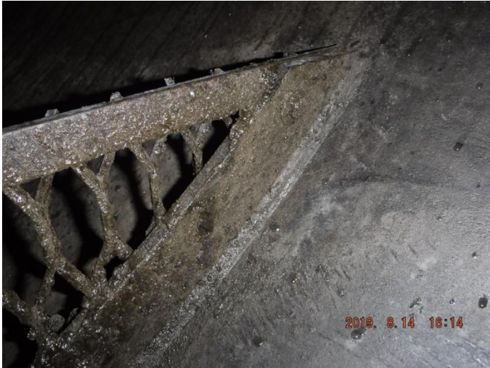
Typical Weir to Shell Weld
