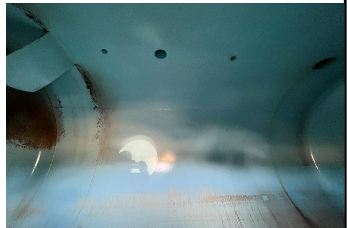
Internal view of head and shell surface. (Sludge on shell & upper head)
