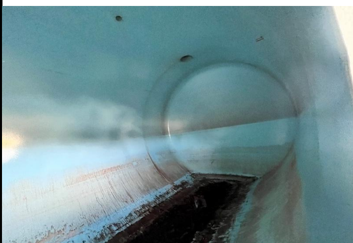
Internal view of lower shell surface. (Sludge residue)
