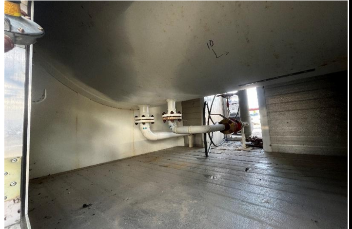
External shell belly view in crawl space.
