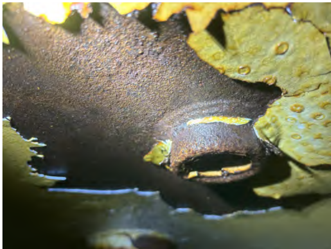
12:00 coating failure
