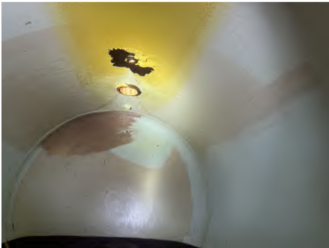
12:00 coating failure
