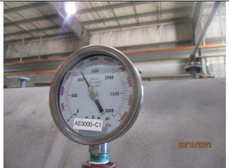
Figure 6: Piping hydrotest at 1100 psi Gauge AE 3000-C1
