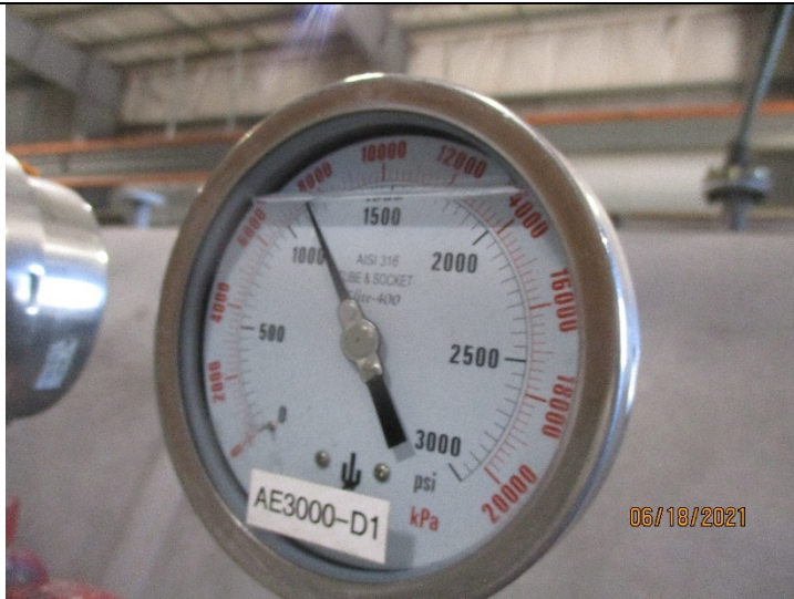
Figure 5: Piping hydrotest at 1100 psi Gauge AE 3000-D1
