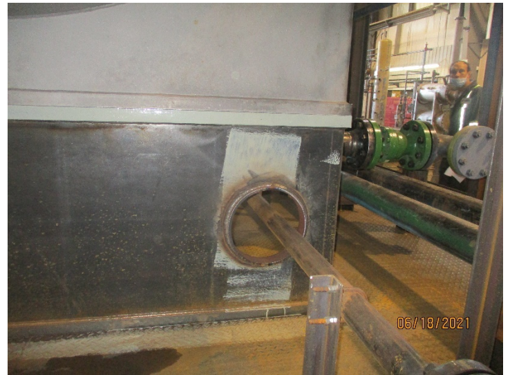
Hole is 8 inch diameter with a 0.375" wall reinforcement
