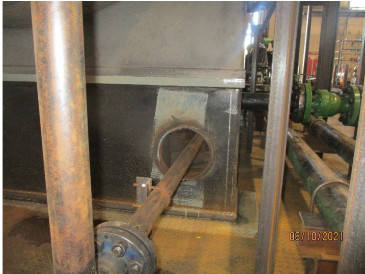
Hole thru saddle support, Aspire to confirm load bearing ability of saddle with full hydrotest weight
