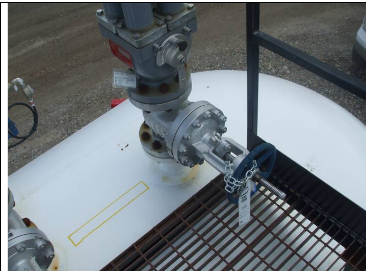
PSV location – B/V Locked open
