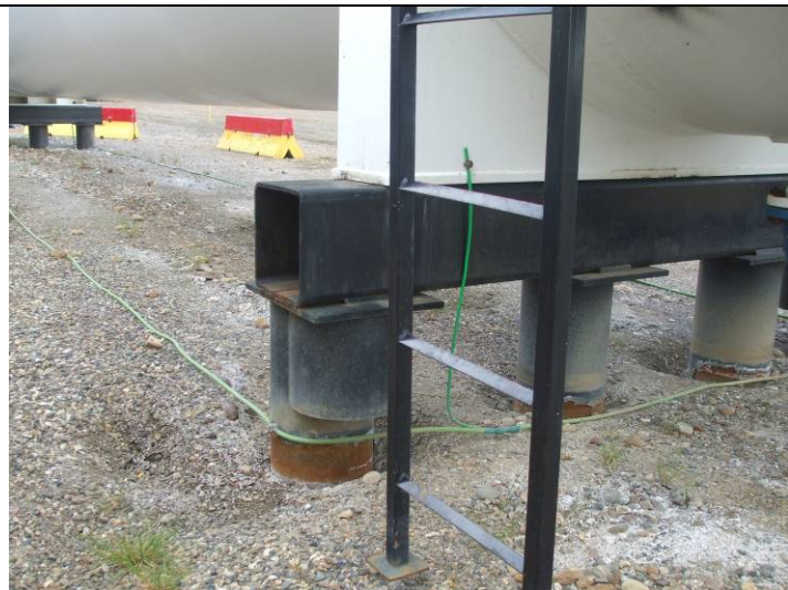
Grounded – Skirt & Piling
