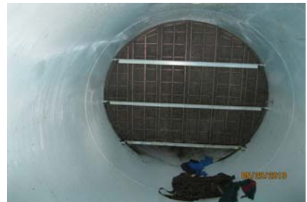
Demister is raised 12" off of floor, is secure and in good shape
