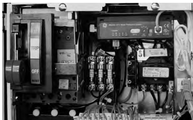
Figure 40. Fuse location.
