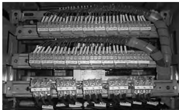
Figure 19. Typical Type C terminal board at the top of a section
