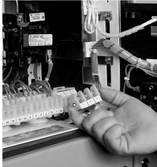
Figure 22. Mounting the terminal block
