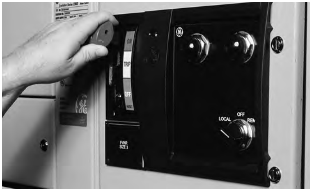
Figure 29. The door cannot be opened when the disconnect is ON.
