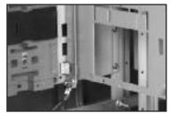
(Optional) Vertical copper ground bus allows direct grounding of unit saddles to the equipment ground bus. A unit ground bus stab engages the vertical ground bus before the unit power stabs engage the vertical bus. A load ground lug is available for customer cable grounding. Termination points are located at the rear of the bucket, next to starter.
