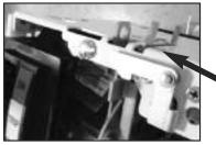
AFM units utilize a mechanical stab interlock on the top of the unit to prevent inserting the unit into the enclosure while the unit stabs are extended.
