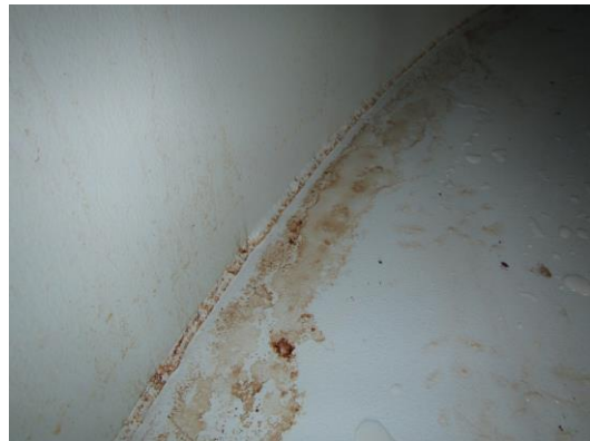
FLOOR TO SHELL FILLET WELD
