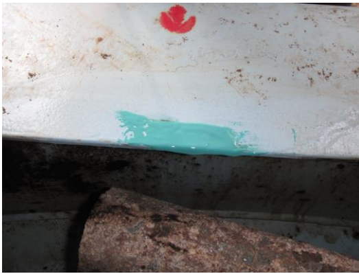
MANWAY COATING REPAIR
