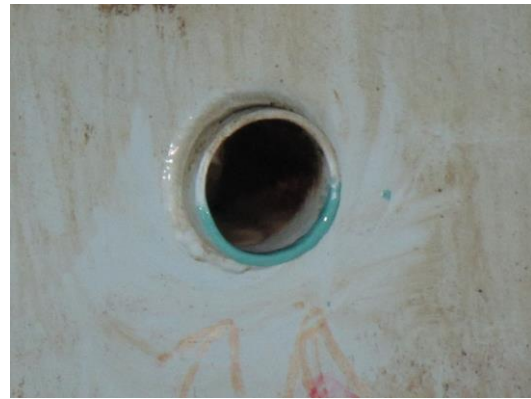
NOZZLE COATING REPAIR
