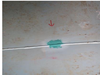
FLOOR LONGSEAM COATING REPAIR
