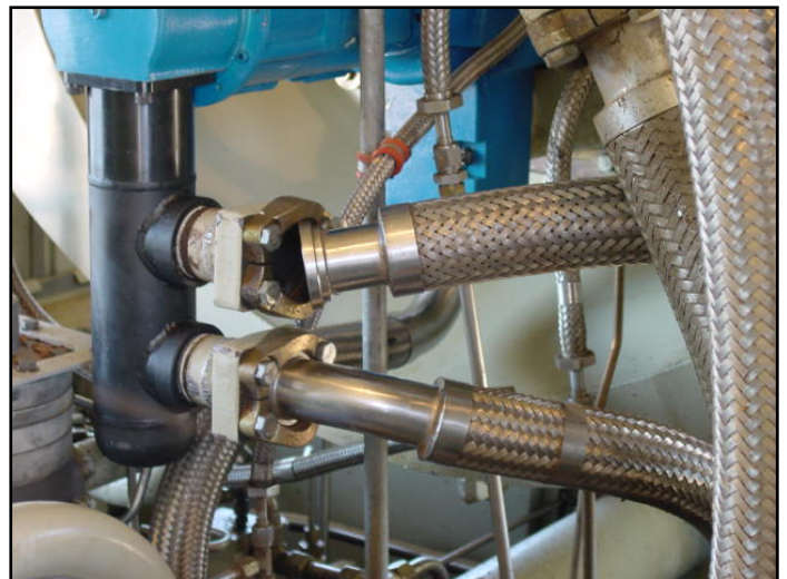
Figure 8. Exhaust Hose Installation
