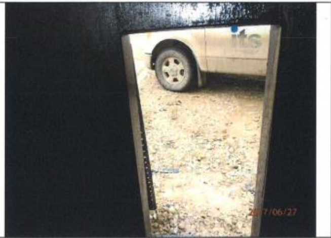
Internal Manway Overview
