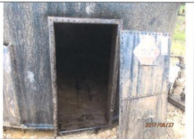
External Manway Overview
