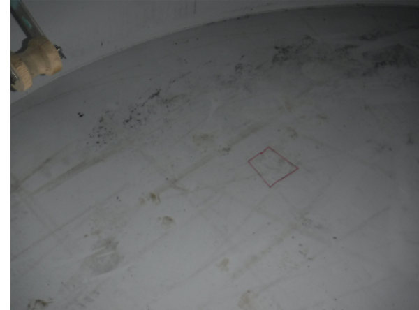
Floor patch area found with MFE scan 12" Diameter
