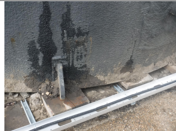
Floor to shell water/ mud saturation
