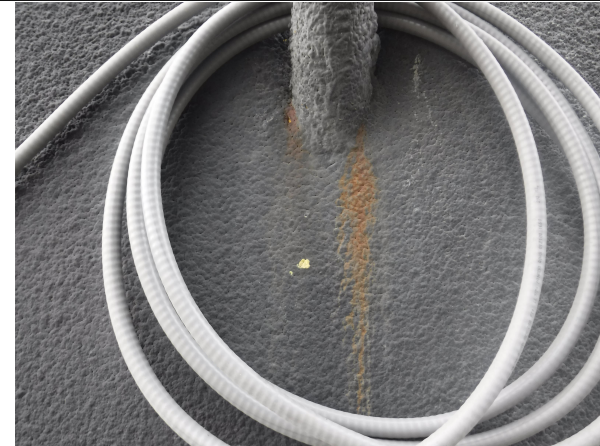
Rust rundown from 2" Scada
