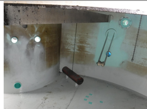
Internal float missing guide wires
