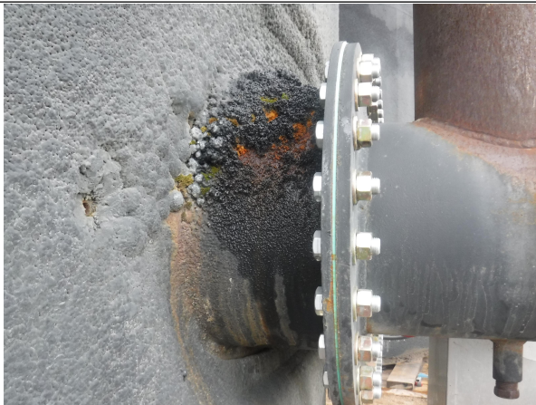
Moss Growth and rust rundown from firetube throat
