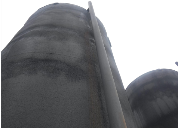
Rust rundown from Gauge board clips
