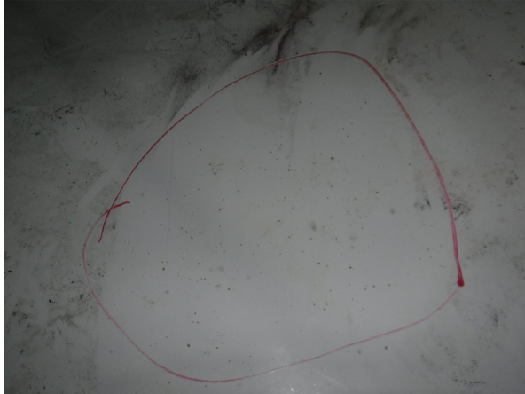
Burnt coating area on the floor
