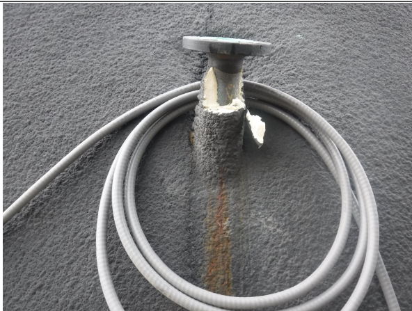
Rust rundown from 2" Scada
