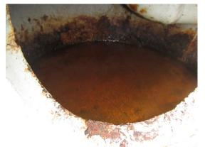
GAS OUTLET THROUGH ROOF SEAL FAILURE
