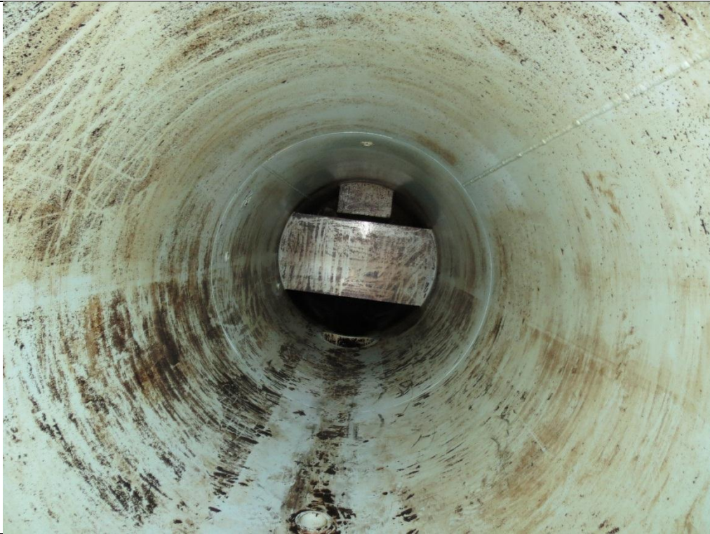
General Internal View From the East End
