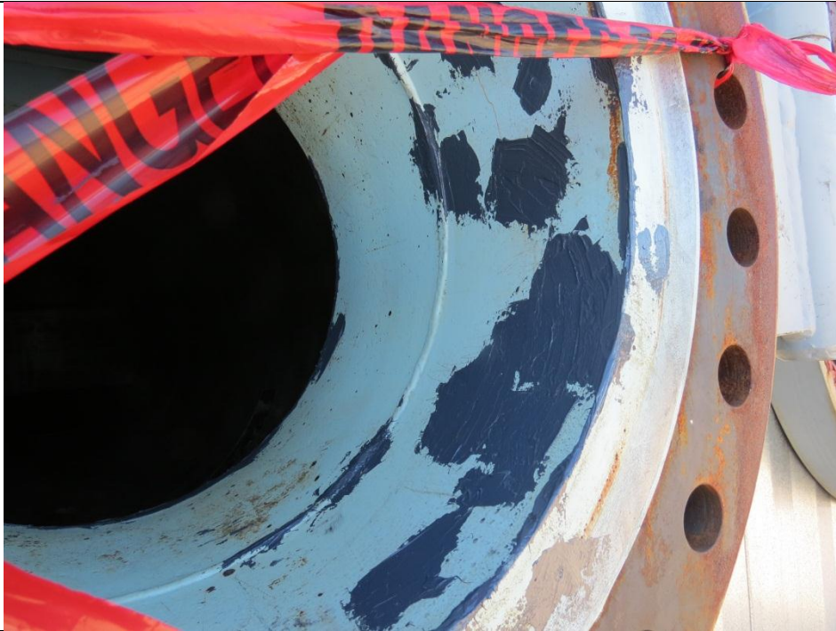
Coating Repairs inside Manway
