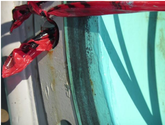
MANWAY NOZZLE COATING REPAIR
