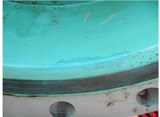
MANWAY NOZZLE COATING REPAIR
