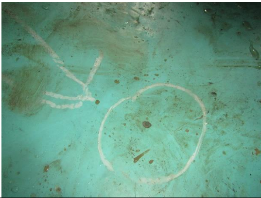
BOTTOM SHELL SMALL COATING FAILURE
