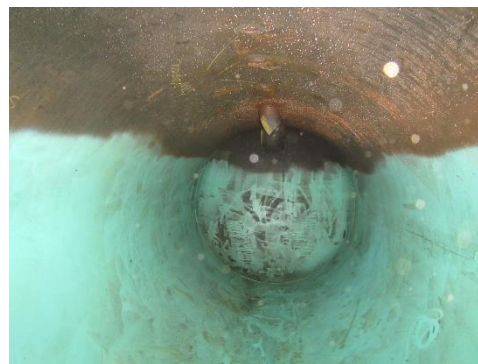
INTERNAL OVERVIEW - BOTTOM 2/3 OF VESSEL COATED
