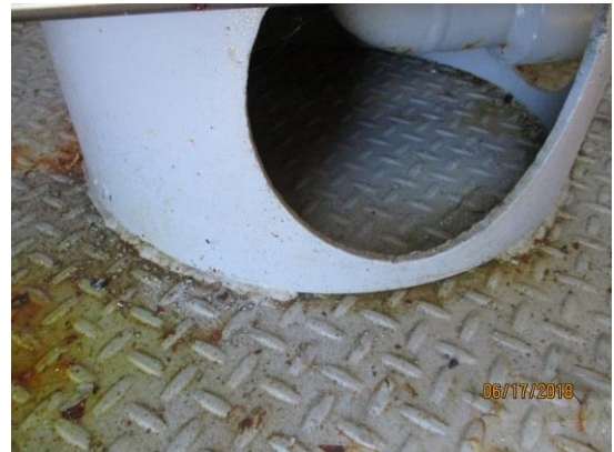
Skirt welded to floor
