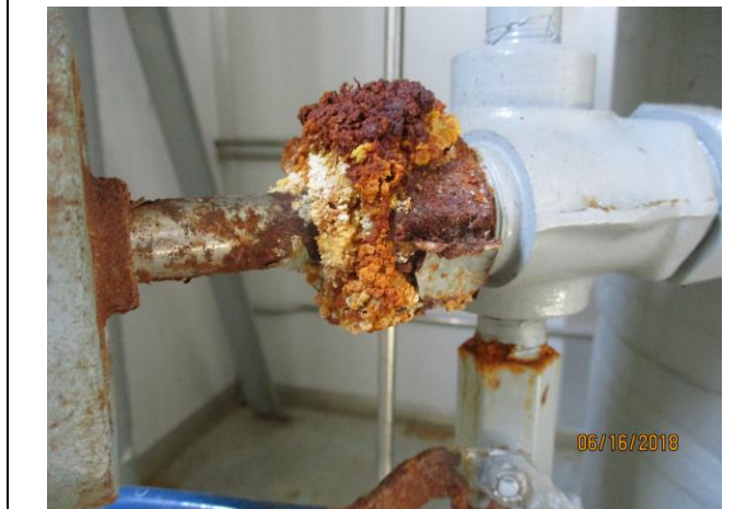
Leaking sight glass connection (TYP)
