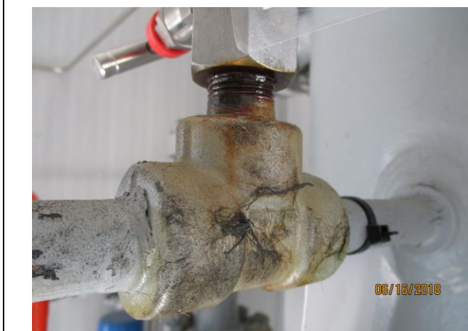
Leaking instrument connection
