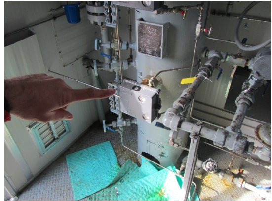
There is product buildup indicating a leak from fisher control to shell threaded connection.
