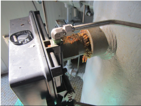
There is product buildup indicating a leak from fisher control to shell threaded connection.
