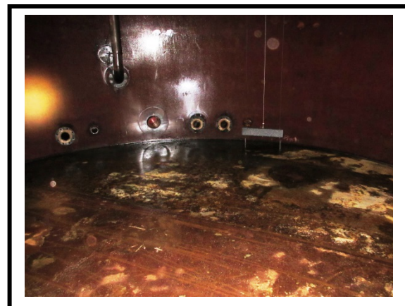
Overall floor & internal nozzles. No pitting or corrosion found.
