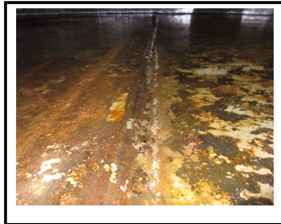
Floor lap joint fillet weld.
