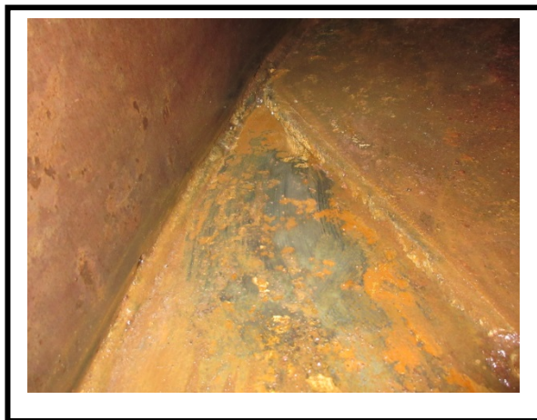
Surface scale scraped away leaving smooth original plate finish.
