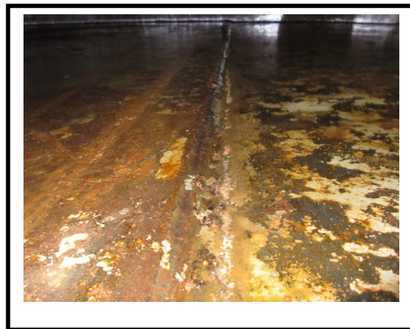
Floor lap joint fillet weld.
