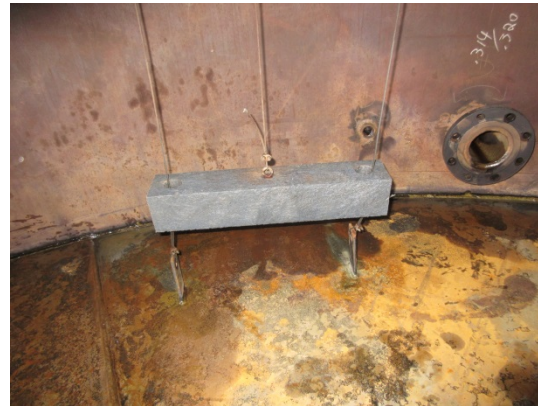
Level indication in good condition. Composite float moves freely within guide cables.
