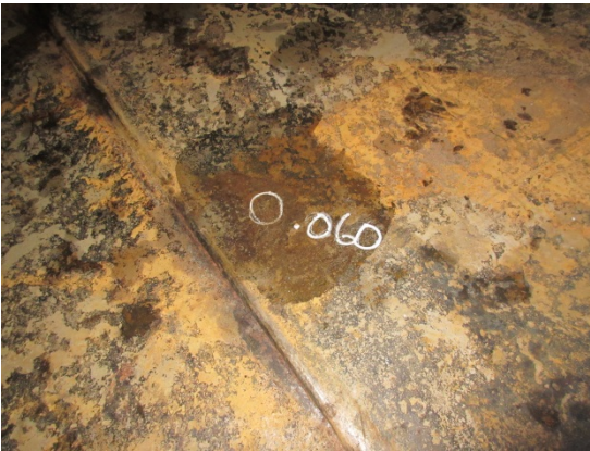
Random clusters of pitting throughout floor plate at 0.020" – 0.060" in depth.
