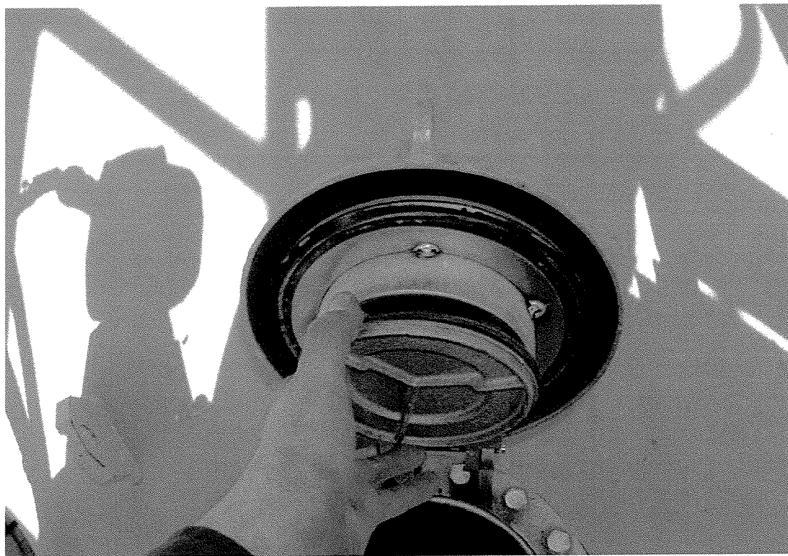
Photo #16: Fully functional vacuum breaker
