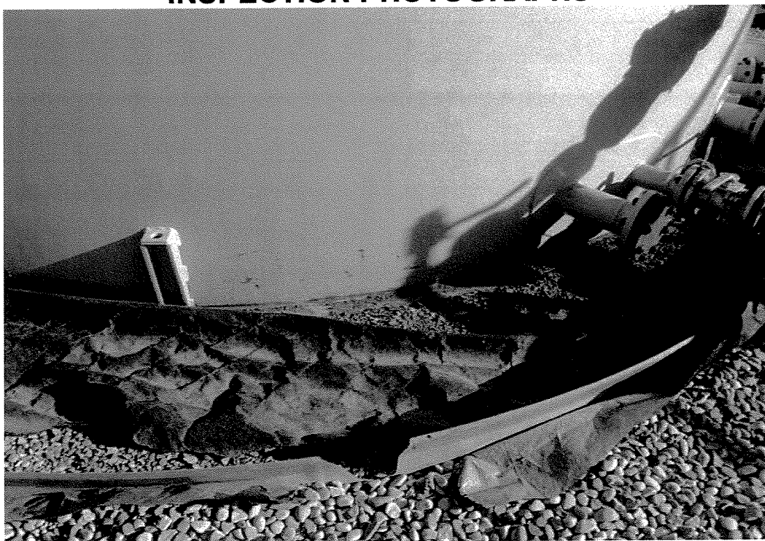
Photo #17: Soil piled up around shell bottom, anchor points not utilized
