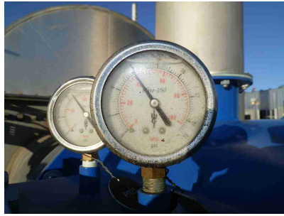
Pilot PRV pressure gauge
