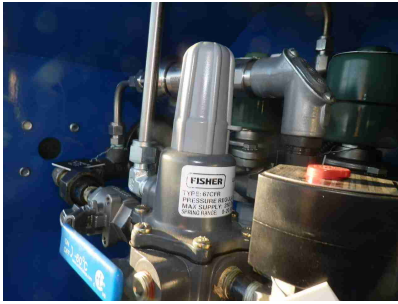
Pilot pressure regulator - PRV
