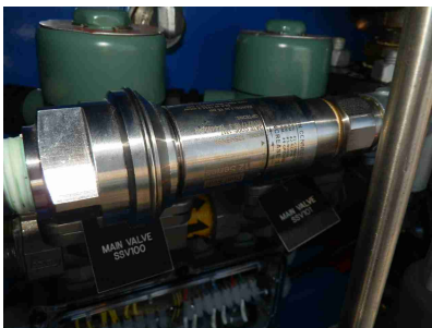
Low pressure shutdown - PSLL
