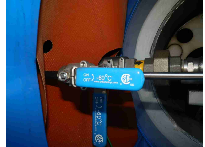
Pilot burner test firing valve
