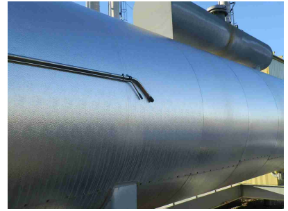
Vent line terminations
