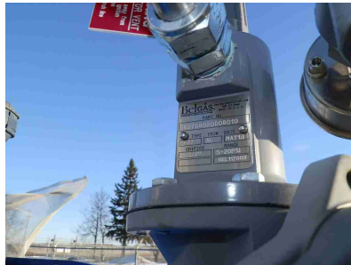
Main fuel pressure regulator - PRV
