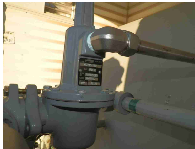
Upstream PRV - main fuel inlet pressure
