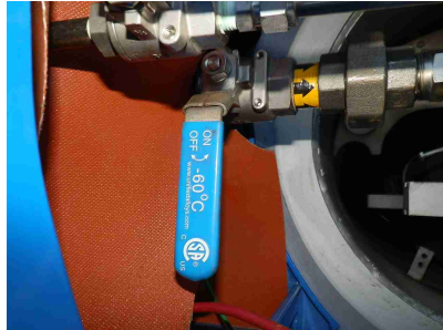
Main burner test firing valve
