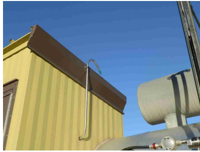
Vent line terminations
