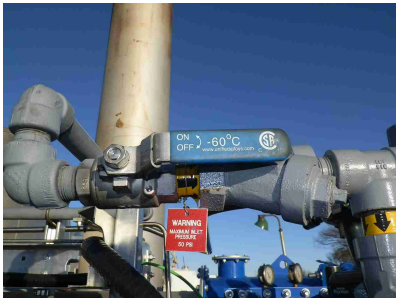
Main fuel manual shutoff valve and y-strainer
