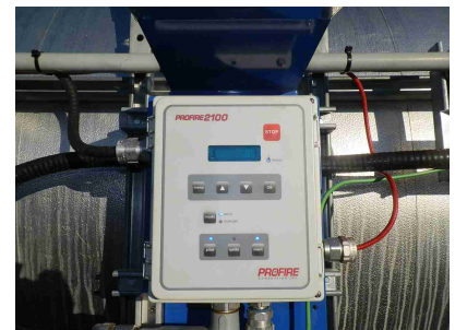
Burner Management System - BMS
