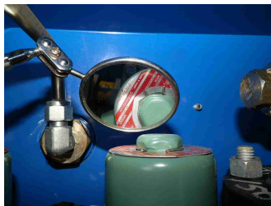
Main fuel safety shutoff valve - SSV
