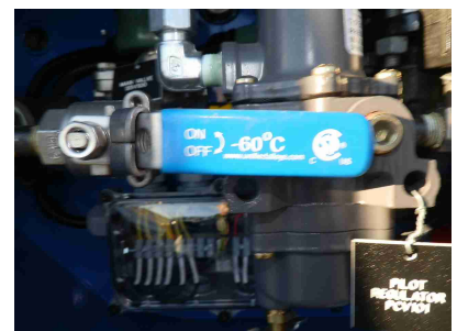
Pilot manual fuel shutoff valve
