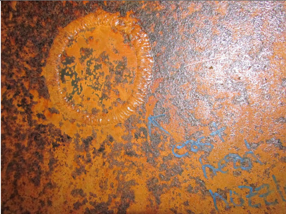
Nozzle has been removed in east head
