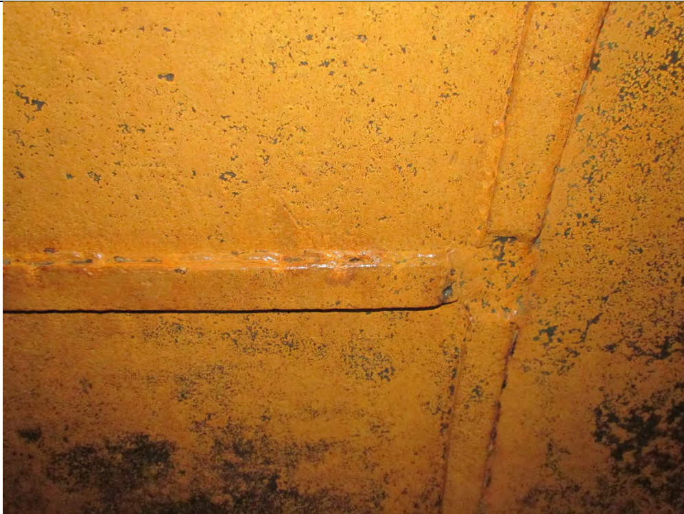
Backing plates for weld seams
