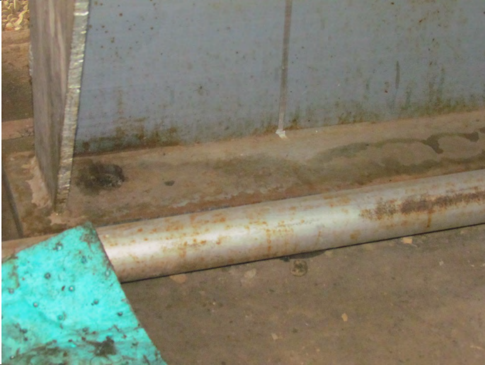
Missing anchor bolts and cement foundation
