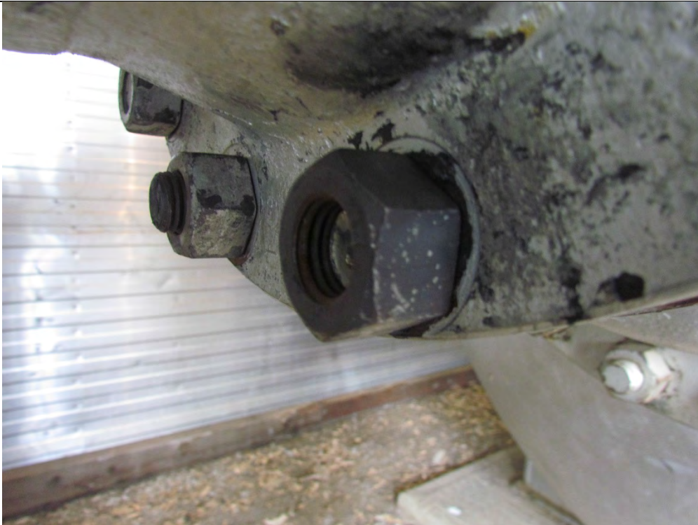
Short bolting on inlet nozzle
