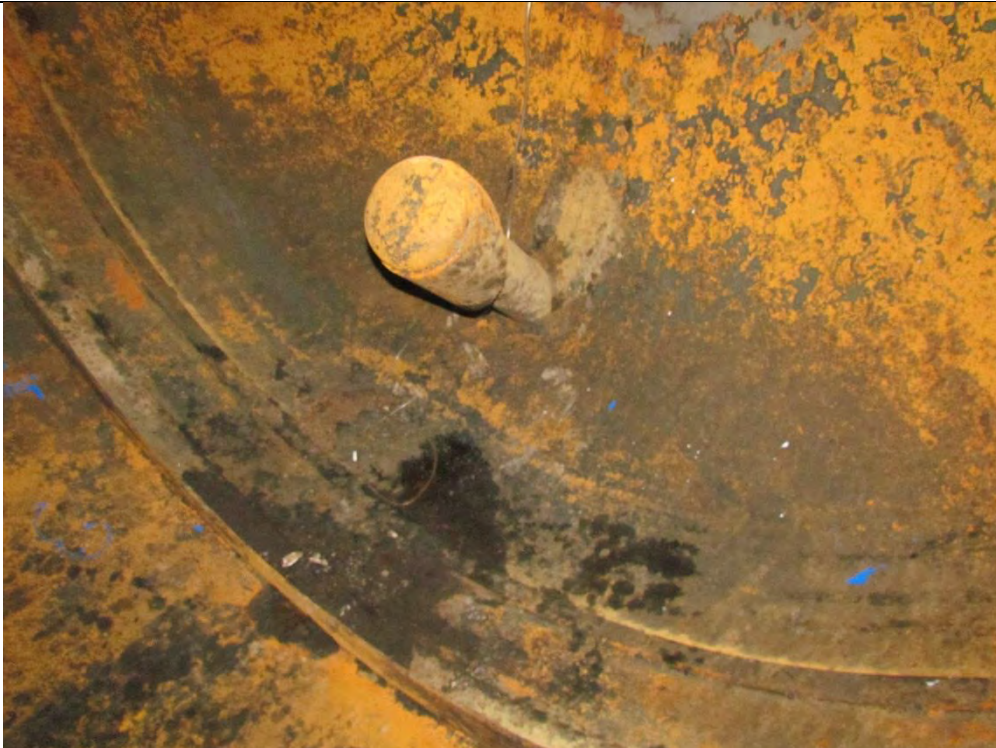
Internal vessel pipe and backing plate at west head
