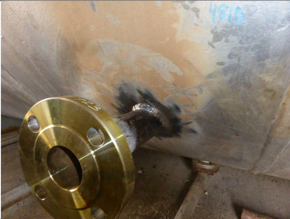
General view of completed weld (1)
