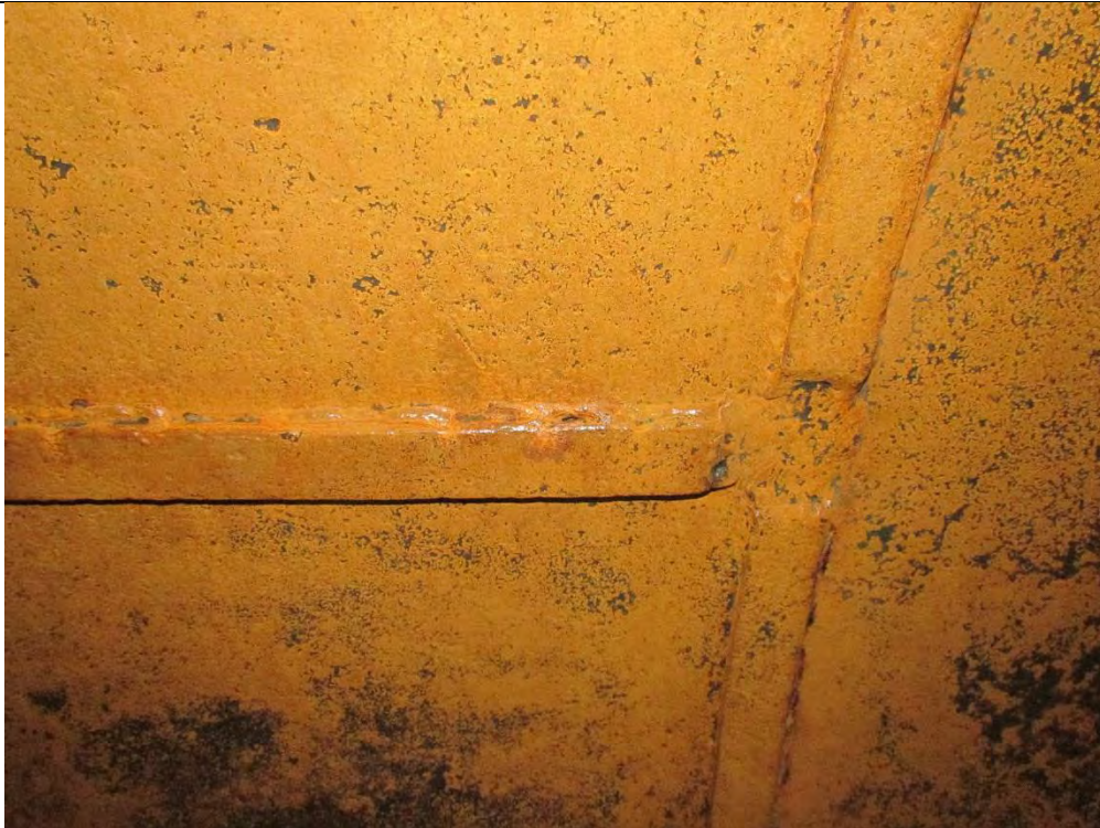
Backing plates for weld seams
