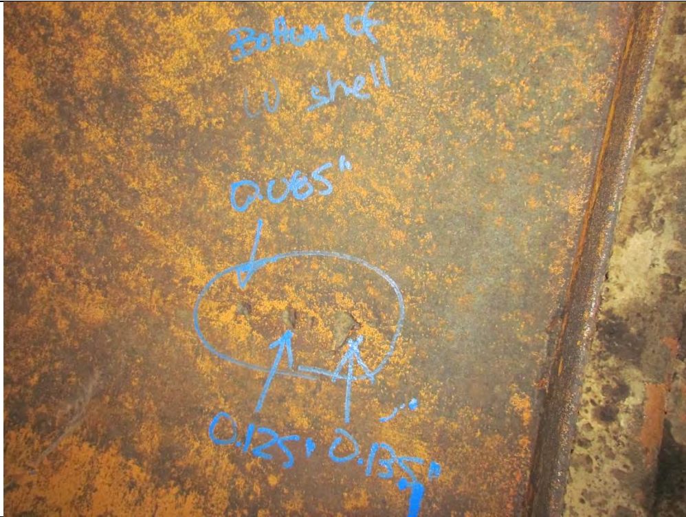
0.065"/0.125"/0.135" plate defects in bottom of west end of shell
