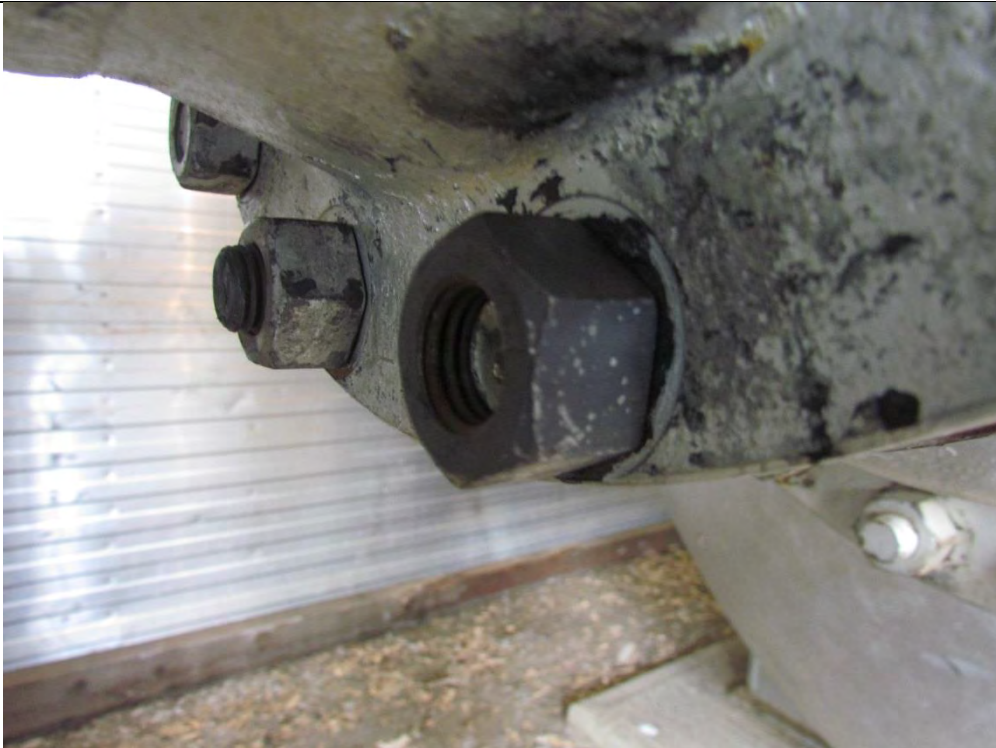
Short bolting on inlet flange
