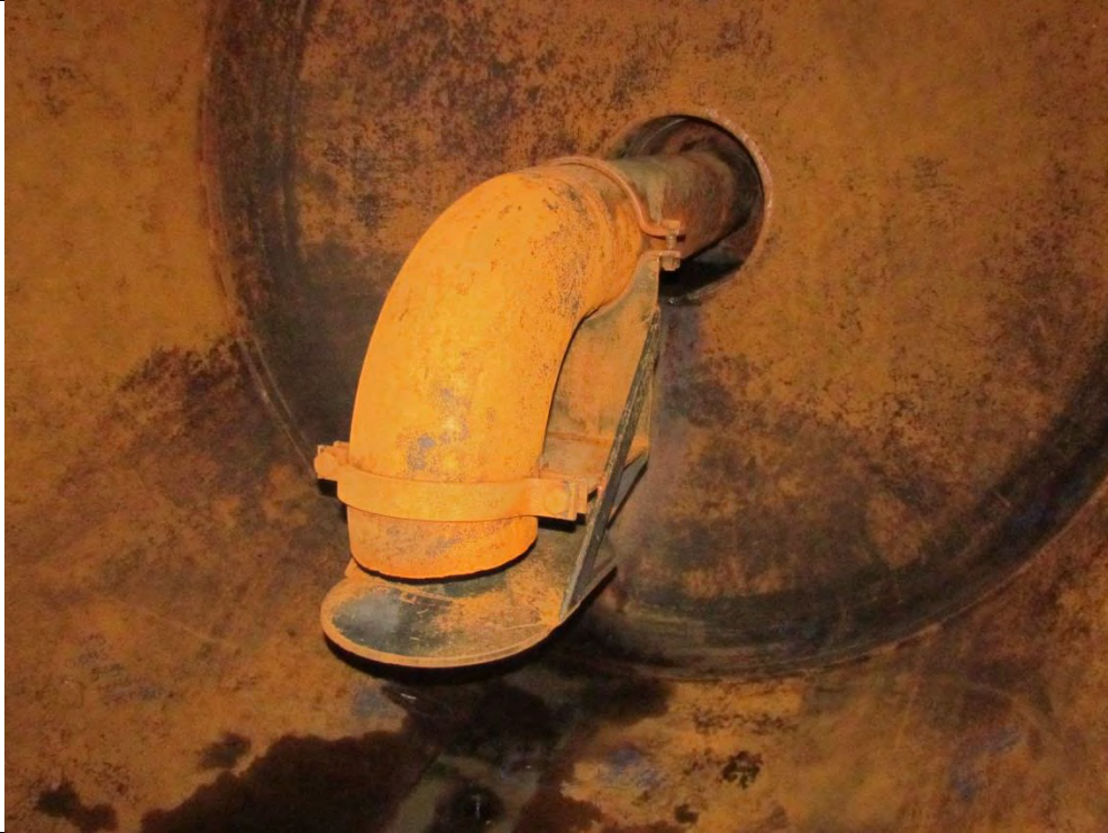
Vessel inlet piping and deflector plate assembly
