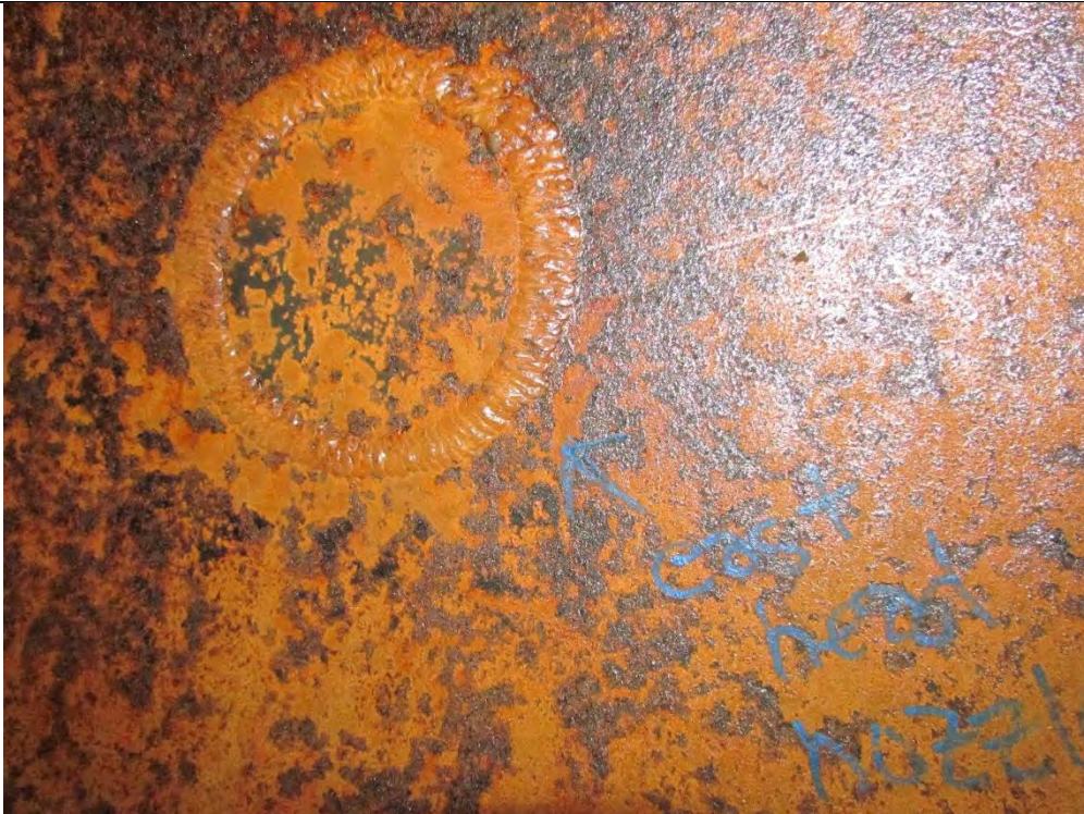
Nozzle has been removed in east head
