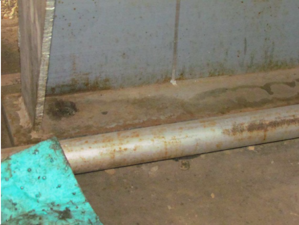
Missing anchor bolts and concrete foundation
