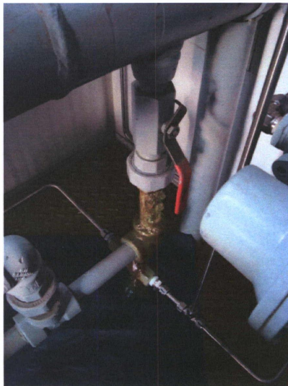
Active Leaks in Threaded Fittings
