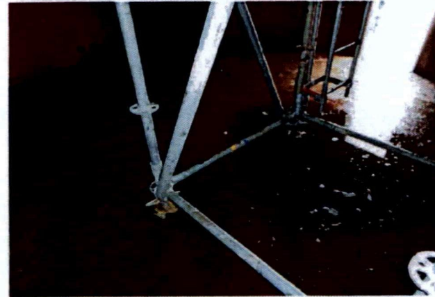
43 FLOOR READINGS & 10 SHELL READINGS TAKEN LOW FLOOR READING: 0.234" LOW SHELL READING: 0.237"
