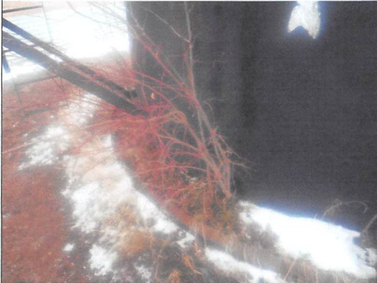
Trees growing from the base, recommend lifting the tank and resetting the base
