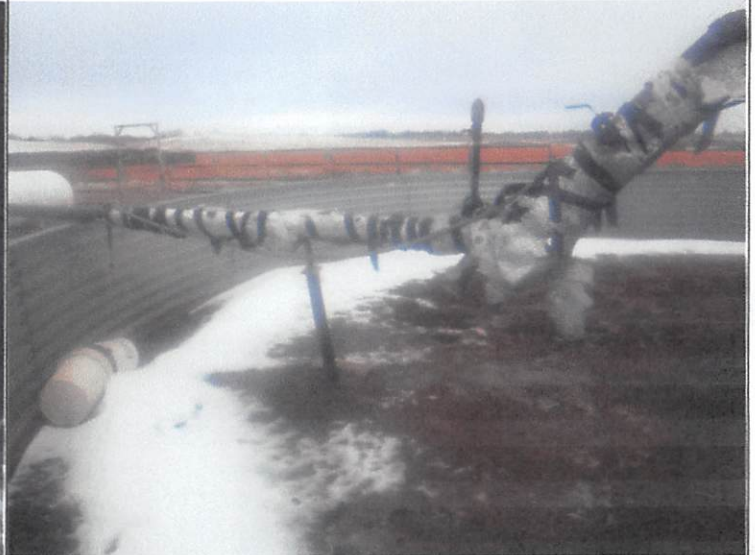
straighten out the flow line stands
