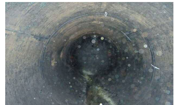
CAN TO CAN CIRC WELD T INTERSECTIONS
