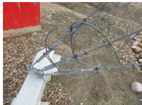
Guy Wire turnbuckles and support
