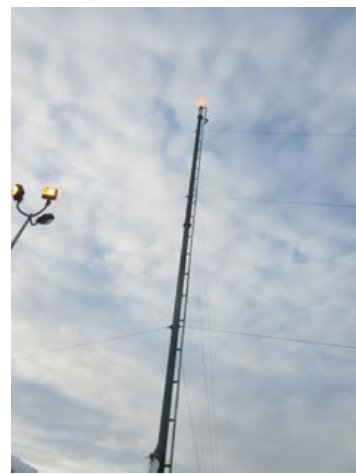
Overall View upper part of stack
