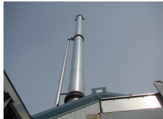
OVERVIEW ABOVE ROOF
