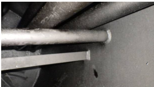
Coil support bracket
