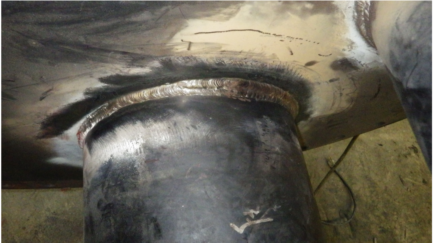
Outside Fillet Weld – 8 Inches Long
