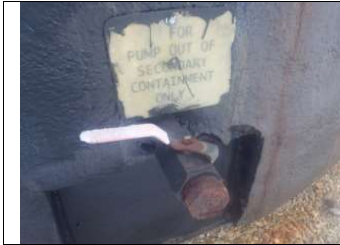
Secondary containment drain
