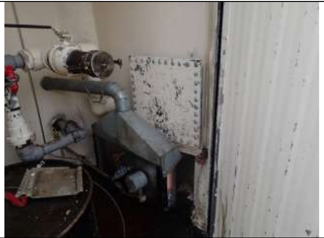
Interior of attached shack. Interstitial space leak indicator to right of manway.
