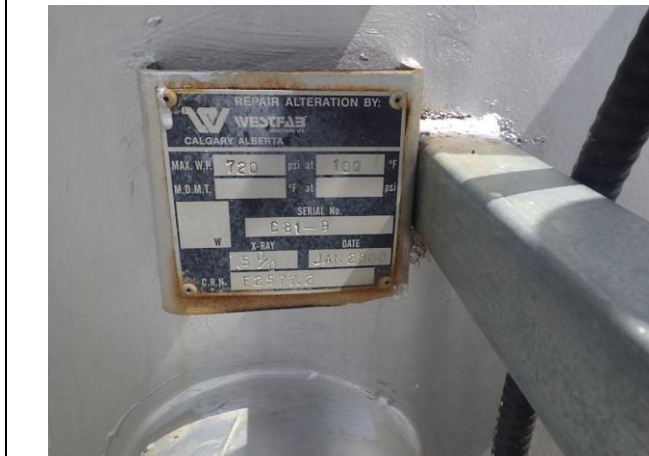
VESSEL ALTERATION PLATE
