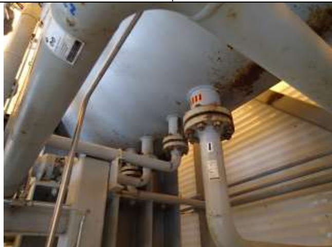
Drain piping/bottom shell
