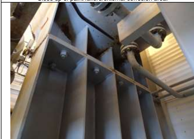
Support system at manway end photo 2
