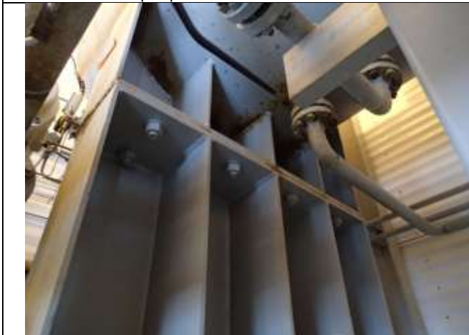
Support system at manway end photo 2
