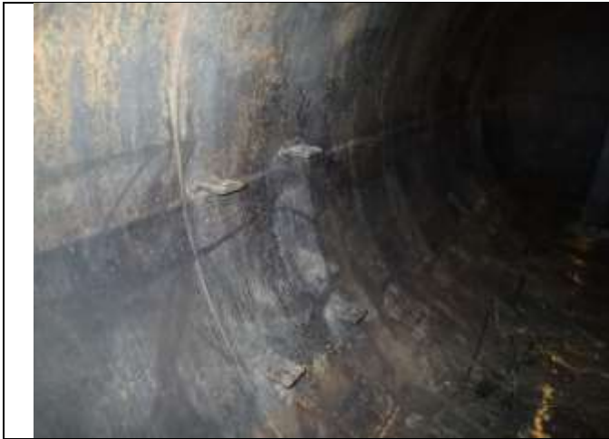
May 2017 Internal – left side shell and vein pack support clips
