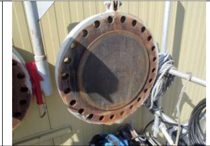
May 2017 Internal – Manway cover
