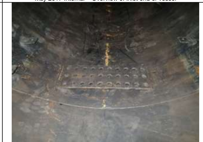
May 2017 Internal – mid lower shell and vein pack support
