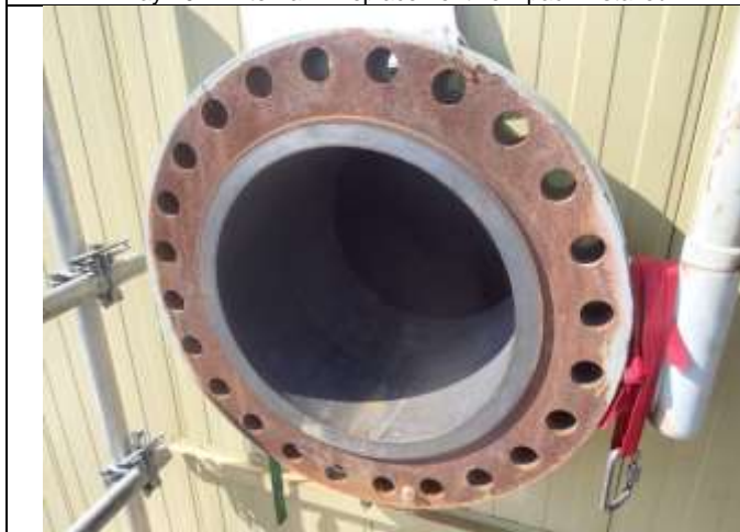
May 2017 Internal – Manway face and nozzle neck
