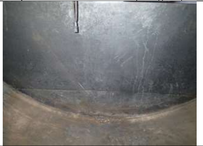
May 2017 Internal – Inlet side of weir
