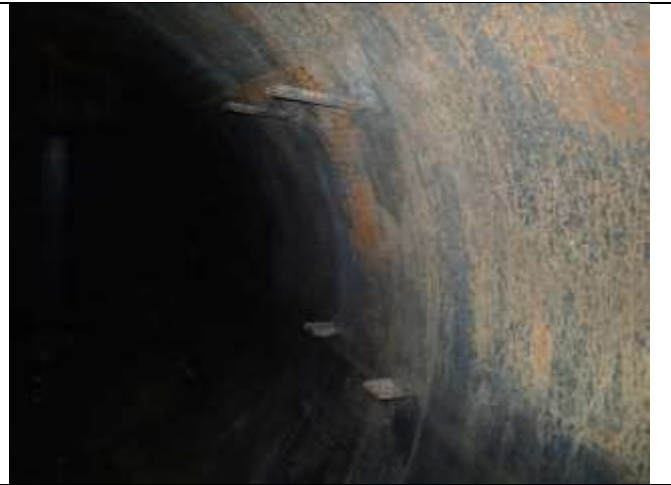
May 2017 Internal – left side shell and vein pack support clips
