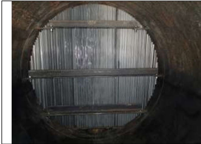
May 2017 Internal – Replacement vein pack installed
