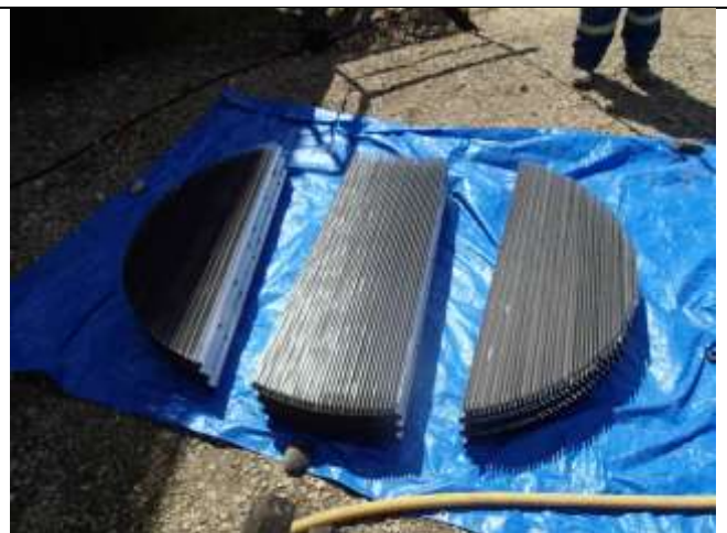
May 2017 Internal – New replacement vein pack prior to installation
