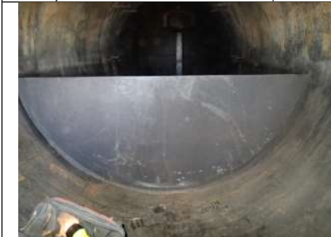
May 2017 Internal – Outlet side of weir and lower shell
