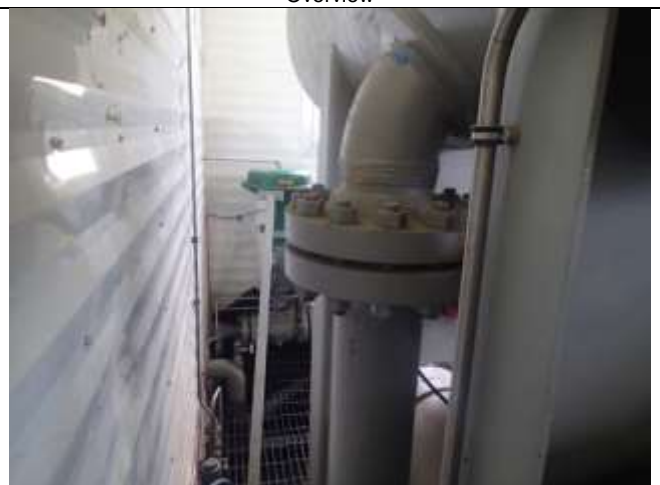
Outlet piping to blowcase
