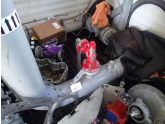
PSV overview – location on inlet to slug catcher
