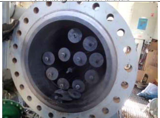
Internal – Access opening showing sealing surface, portions of shell and filter mounting hardware
