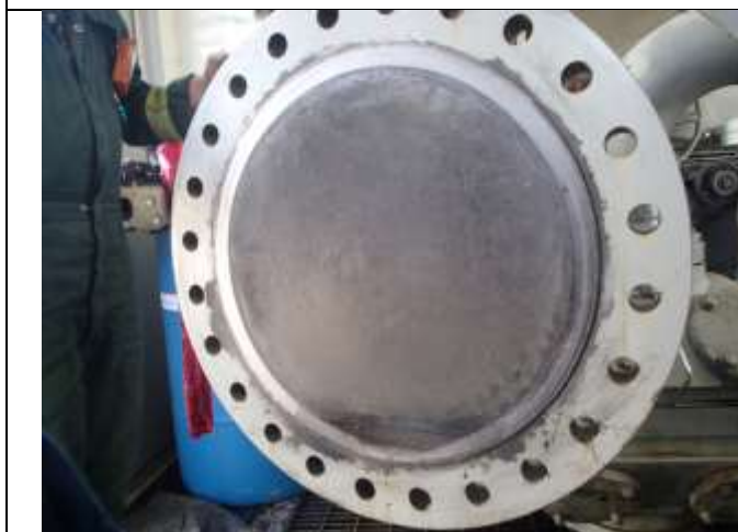
Internal – Access opening cover flange
