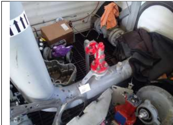
PSV overview – location on inlet to slug catcher
